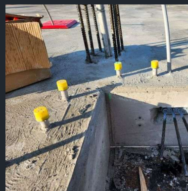
After pour: immediate barrier installation, no scanning or drilling
